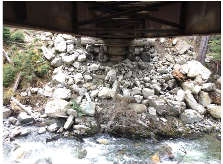
Left Bank Abutment when facing downstream
