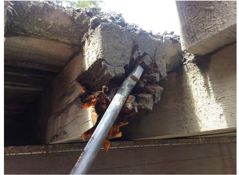
Panel 1 upstream tie condition
