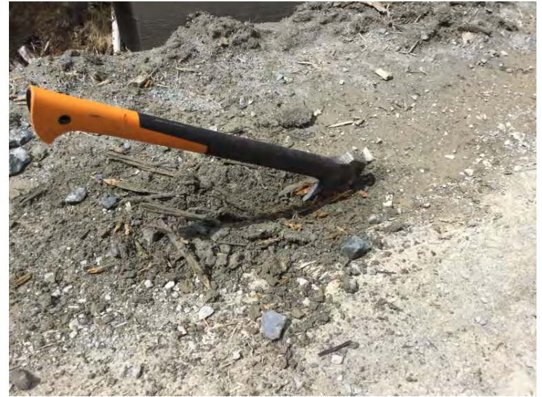
Timber plank condition (Poor) in Panel 5, downstream wheel path
