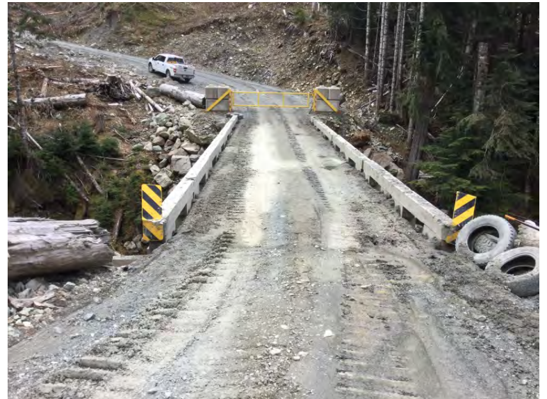
Approach from Right Bank when facing downstream
