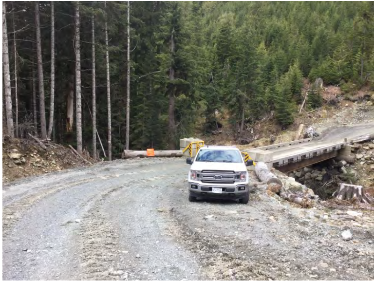
Approach from Left Bank when facing downstream
