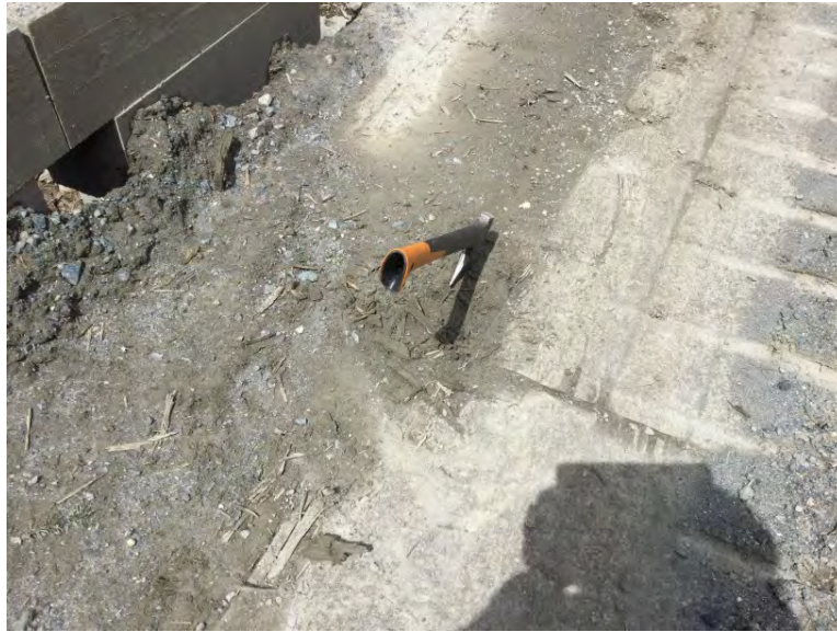
Timber plank condition on Panels 4 and 5 at downstream wheel path location
