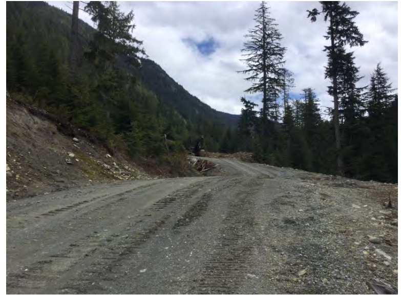
Excavator parked at woods end of bridge
